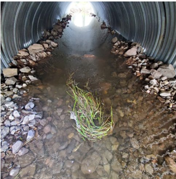
Stream bank simulation rock placement in-progress
